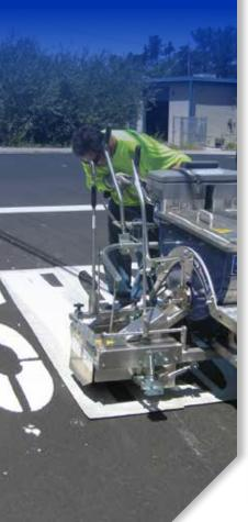
The SmartDie II System is the industry standard in screed box technology—only from Graco. It's innovative design allows users to use it with or without direct heat allowing more flexibility in all weather conditions. The 4-torch die heat system (standard on ThermoLazer ProMelt) allows contractors to optimize and extend their thermoplastic striping opportunities, especially in cooler climates.
