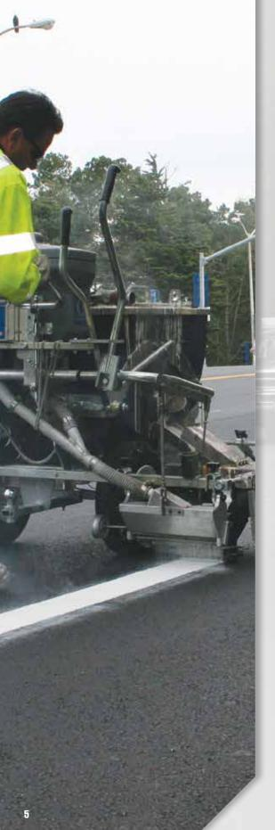
ThermoLazer 300TC Dual **PaddleMax™ System** A single chamber hopper holds 300 lb of hot thermoplastic material, reducing the need to constantly refill.
